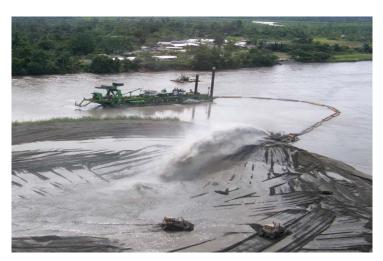
OTML has continuously engaged the CSD 'Cap Martin' through Dredging International's local entity Dredeco PNG since the start of the program in 1998, to operate and capture the possibly polluted sand-sized sediments flowing down the river, and thereafter store them in engineered stockpiles on the East and West riverbanks of the OK TEDI river at Bige. To date, over 170 million m3 of sediments have been removed and pumped in stockpiles up to 30 m high, situated up to 6 km from the dredging area.
